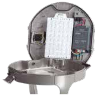
Automatic electric disconnection
